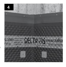
■ Do not install DELTA®-FAST'ners within 3" (8 cm) of outside corners to avoid damaging the concrete.
