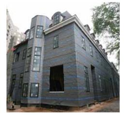
It is well known that moisture can be a major source for trouble in construction. In building envelopes and wall cavities moisture can cause mold, mildew, and major decay, whether the origin of moisture is rainwater that passes the exterior cladding, or condensing vapor from the interior. DELTA®-DRY provides a unique approach to manage both moisture from inside and outside in order to protect the wall cavity against moisture damage.
